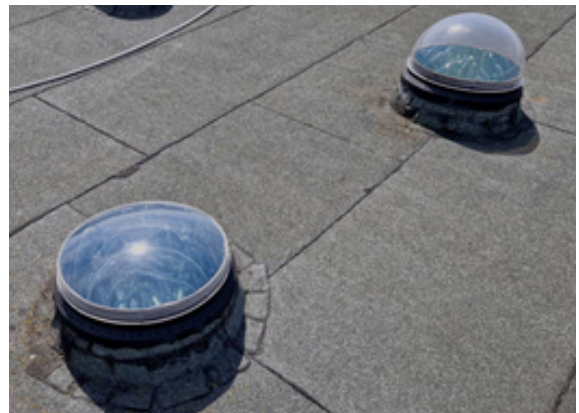
Tubular daylighting devices must be measured and rated per ANSI/NFRC 203 standard.
