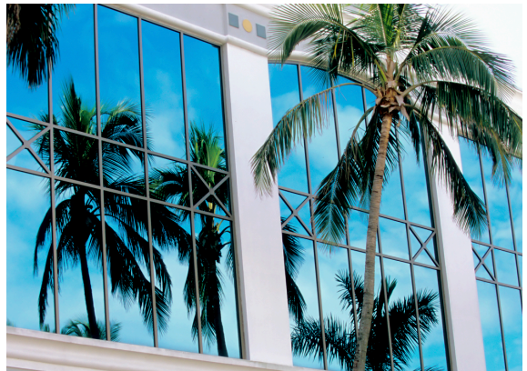
New fenestration products, replacing existing ones, must meet U -factor and SHGC requirements.
